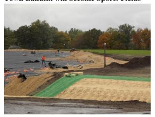
The Town of Amesbury, MA has long had an eyesore, a former landfill visible from I-495 along Hunt Road. Phase one of a transformation towards sports fields will be completed this fall. Charter Environmental was contracted to create a 2% grade on which sports fields will be built in phase two as well as cap the landfill and establish a lush stand of vegetation. This required
